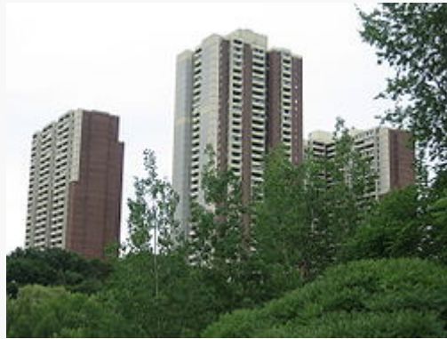
Three of Crescent Town's buildings towering over the Taylor Creek ravine.
